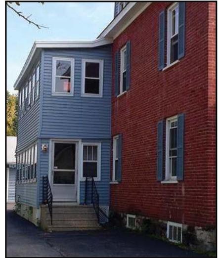
Material change between brick and clapboard made at appropriate structural location.
