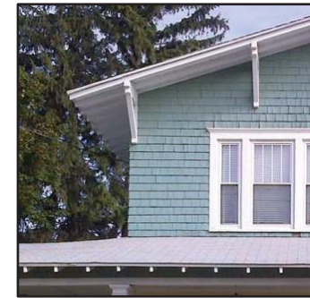
Pitched roof with large overhang, brackets, and exposed rafter tails
